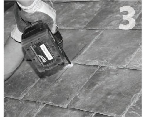
Using a masonry drill bit, drill a pilot hole at the center of the QBBase location you marked in step 2. This drill bit should match the size of the guide bit of your hole saw.
